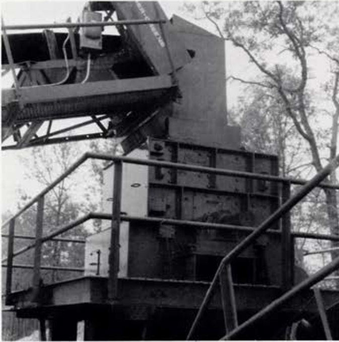
56 FT operating in a load out
